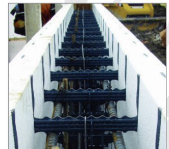
Showing HV Clips holding down a top row that has been cut down to +/- 8" in height
