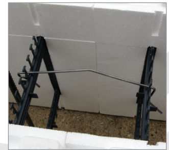
Horizontal Clips in Place
