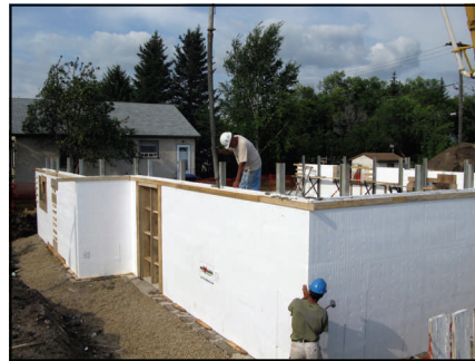
1_4A Fox Blocks Foundation
